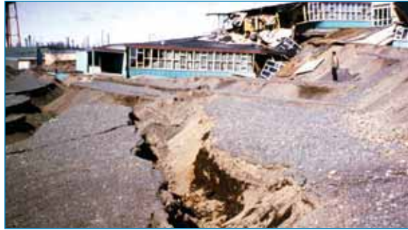
The Government Hill Grade School was destroyed by a landslide during the 1964 Alaska earthquake.
