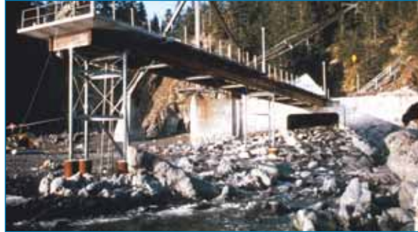
The ground under this dock on Hinchinbrook Island, Prince William Sound, rose about 8 ft during the 1964 Alaska earthquake.
