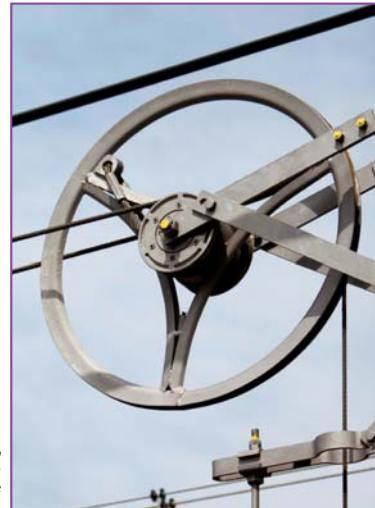
Cable and pulley arrangement used alongside railroad tracks.
