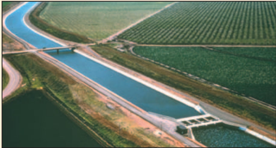
Figure 7 This aqueduct in southern California carries much needed water over long distances.
